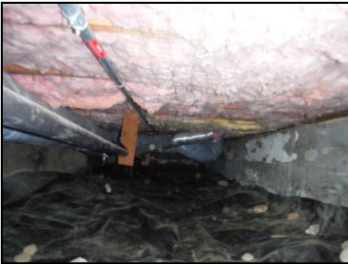
Partial view of the crawlspace under the addition.
