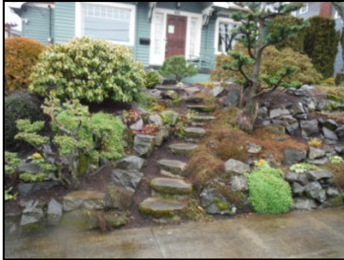
The lack of a handrail on the front stairs could be a fall hazard.
