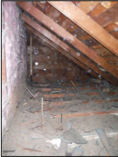
Partial view of the NE eave space.
